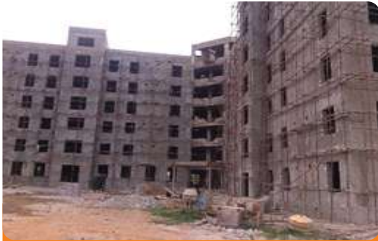
Project: Liberty Suite and Apartment Location: Plot 1806, Cadastral Zone, B13, Gaduwa Estate Scope: Firefighting, Wet Pipe Sprinkler, Hose reel, Fire Hydrant FM200, Dry riser System. PABX, Data and Networking, Hotel Lock, CCTV, PABX and Public Address System
