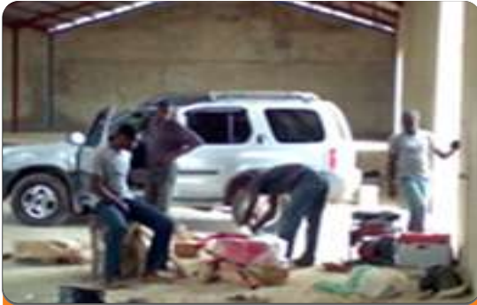
Project: Match Factory Location: Starcase Nig. Ltd. Idu Industrial Estate, Abuja. Scope: Fire Detection and Alarm, Firefighting Installations
