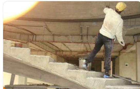
Project: Office Complex, Ryte Cas Location: Wuse II, Abuja. Scope: Fire Detection & Alarm System, Wet Pipe Sprinklers, Wet Riser, Dry Riser & CCTV System
