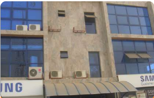
Project: Jeff Bamiro Complex Location: Wuse II, Abuja Scope: Fire Detection and Alarm, Wet Sprinkler System
