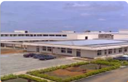
Project: Accident and Emergency Ward Location: Jos University Teaching Hospital, Jos, Plateau State Scope: Fire Detection and Alarm, Firefighting and Installations
