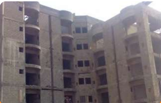
Project: A.M Development Concept Location: Gudu District, Apo, Abuja Scope: Fire Detection & Alarm System, Fire Fighting Installation
