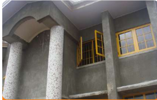
Project: Residential Location: Apo District, Gudu, Abuja. Scope: Conventional Fire Detection & Alarm System, Wet Pipe Sprinkler System.
