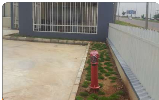
Project: Emadeb Filling Station Location: Kado, Abuja Scope: Fire Fighting Installation
