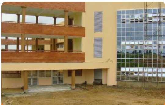
Project: School of Info. & Comm. Technology Location: Federal University of Technology, Minna Scope: Fire Detection & Alarm, Fire Fighting Installation
