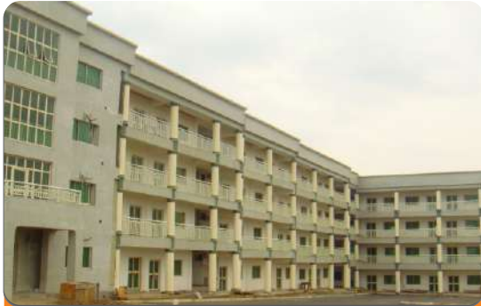
Project: Anbashir Office Complex Location: Utako District, Abuja Scope: Fire Detection & Alarm, Fire Fighting Installation
