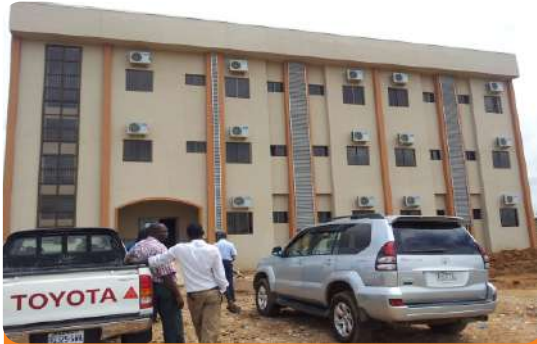
Project: Medical Hostel Location: Jos, University Teaching Hospital Scope: Fire Detection and Alarm Systems
