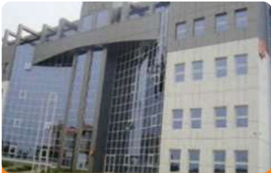
Project: ULO Plaza Location: Wuse, Zone 6, Abuja. Scope: Fire Detection and Alarm
