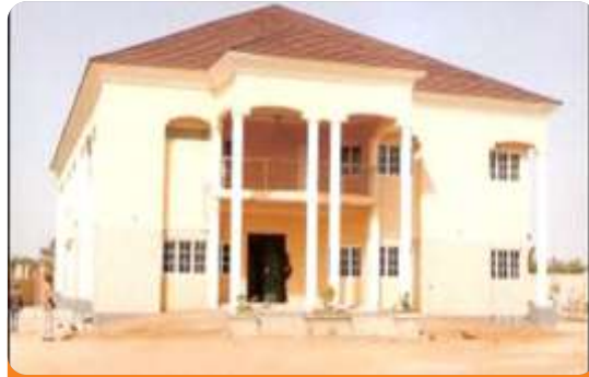
Project: Governor's Lodge Location: Dutse Jigawa Scope: Fire Detection and Alarm, Firefighting and Installations
