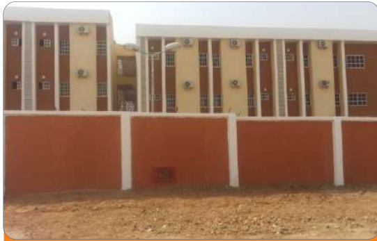
Project: Female Hostel 1 & 2, Block D Location: Federal University of Technology Minna Scope: Fire Detection & Alarm System, Fire Fighting Installation
