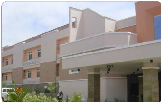
Project: Living Faith Church (Goshen City Guest House) Location: Keffi, Nassarawa Scope: CCTV Surveillance System Installation
