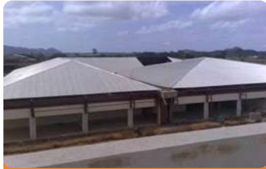
Project: Kitchen and Dining Location: Jos University Teaching Hospital, Jos, Plateau State Scope: Fire Detection and Alarm, Firefighting and Installations
