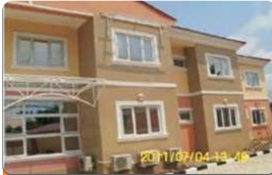
Project: Jabi Luxury Apartment Location: Jabi Luxury Apartment, Jabi, Abuja. Scope: CCTV Surveillance System Installation
