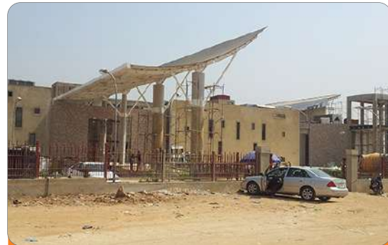
Project: Nigeria Air Force Conference Center Location: Kado District, Abuja Scope: Fire Detection & Alarm System, PABX, CCTV and Surveillance, Public Address System
