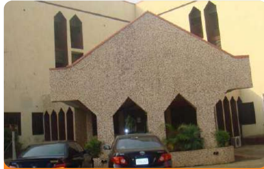
Project: Hotel Mellinnium Location: Wuse, Zone 5, Abuja. Scope: Hotel Lock Management System
