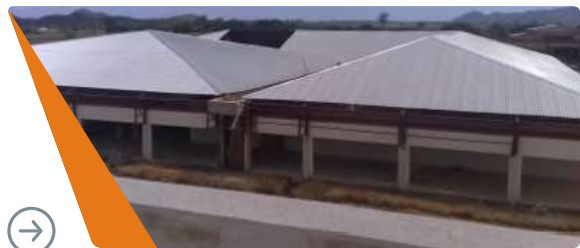
➔ Project: Kitchen and Dinning Location: Jos University Teaching Hospital, Jos, Plateau State Scope: Fire Detection and Alarm, Fire Fighting Installations
