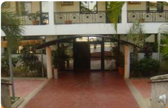
Project: Mediterranean Hotel Location: Asokoro, Abuja. Scope: Hotel Locks Management System
