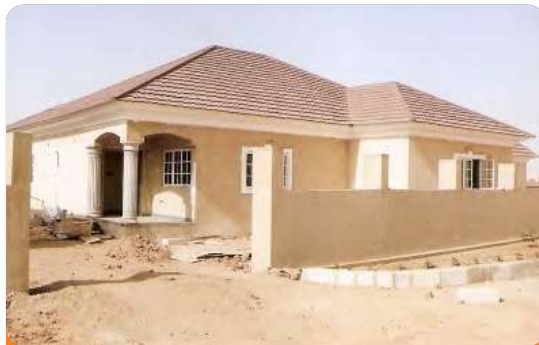
Project: Governor's Lodge Location: Dutse Jigawa Scope: Fire Detection and Alarm System, Firefighting Installations
