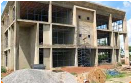
Project: Jeff Bamiro Office Complex Location: Wuse II, Abuja. Scope: Fire Detection and Alarm, Firefighting and Installation
