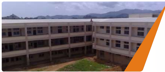
⬆ Project: Operationa Theatre Location: Jos University Teaching Hospital, Jos, Plateau State Scope: Fire Detection and Alarm, Fire Fighting Installations
