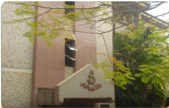
Project: Sharon Regency Hotel Location: Wuse II, Abuja Scope: Hotel Lock Management System
