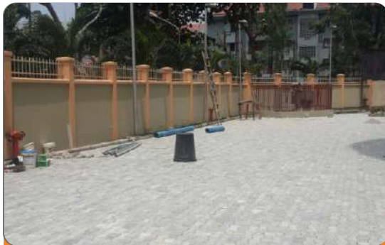
Project: Service Apartments Location: Bourdillion, Ikoyi, Lagos Scope: Fire Detection & Alarm , CCTV, Intruder Alarm PABX, Fire Fighting, Home Automation System
