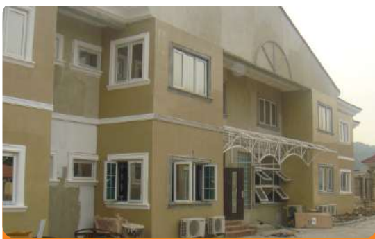
Project: Creation Consult, Service Apartment Location: Jabi, Abuja Scope: Fire Detection & Alarm System
