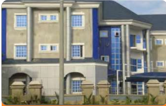
Project: Ta'al Nigeria Ltd Location: Nile Street, Maitama, Abuja. Scope: Fire Detection & Alarm System
