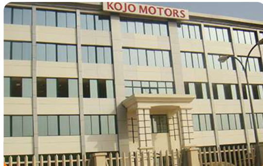
Project: Kojo Motors Location: Utako, Abuja Scope: Fire Detection & Alarm System, Fire Fighting Installation
