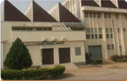
Project: National Institute of Pharmaceutical Research & Development Location: Idu Industrial Layout, Abuja. Scope: Fire Detection & Alarm System
