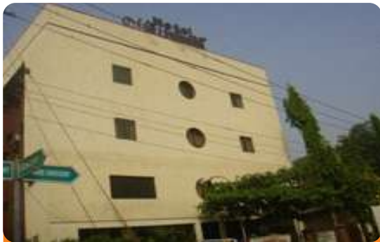
Project: Hotel Millennium Location: Zone 5, Wuse, Abuja Scope: Hotel Locks Management System
