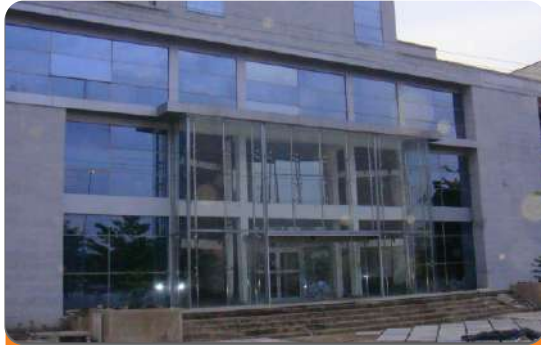
Project: Unit Environmental Office Complex Location: Central Business Area, Abuja. Scope: Fire Detection and Alarm System Installation & Fire Fighting
