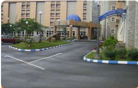
Project: Ibeto Hotels Location: Gudu, Abuja Scope: Fire Detection and Alarm System, CCTV System and External Mechanical Works
